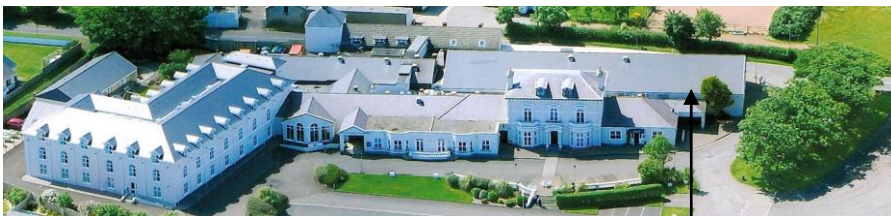
Room Location: Ground Floor behind Magherabuoy House, separate entrance
